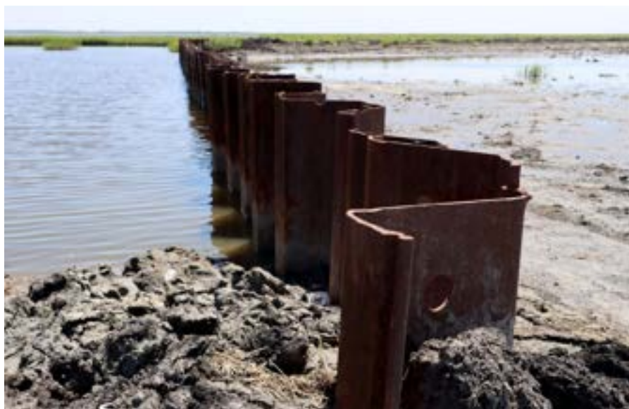
Sheetpile and dikes built for containment cells
