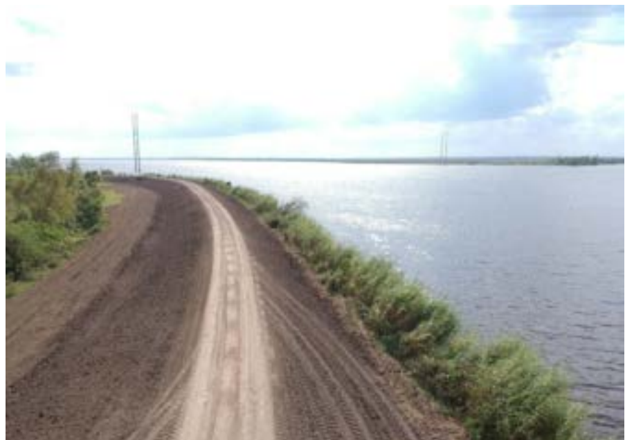
Newly constructed Sunset levee
