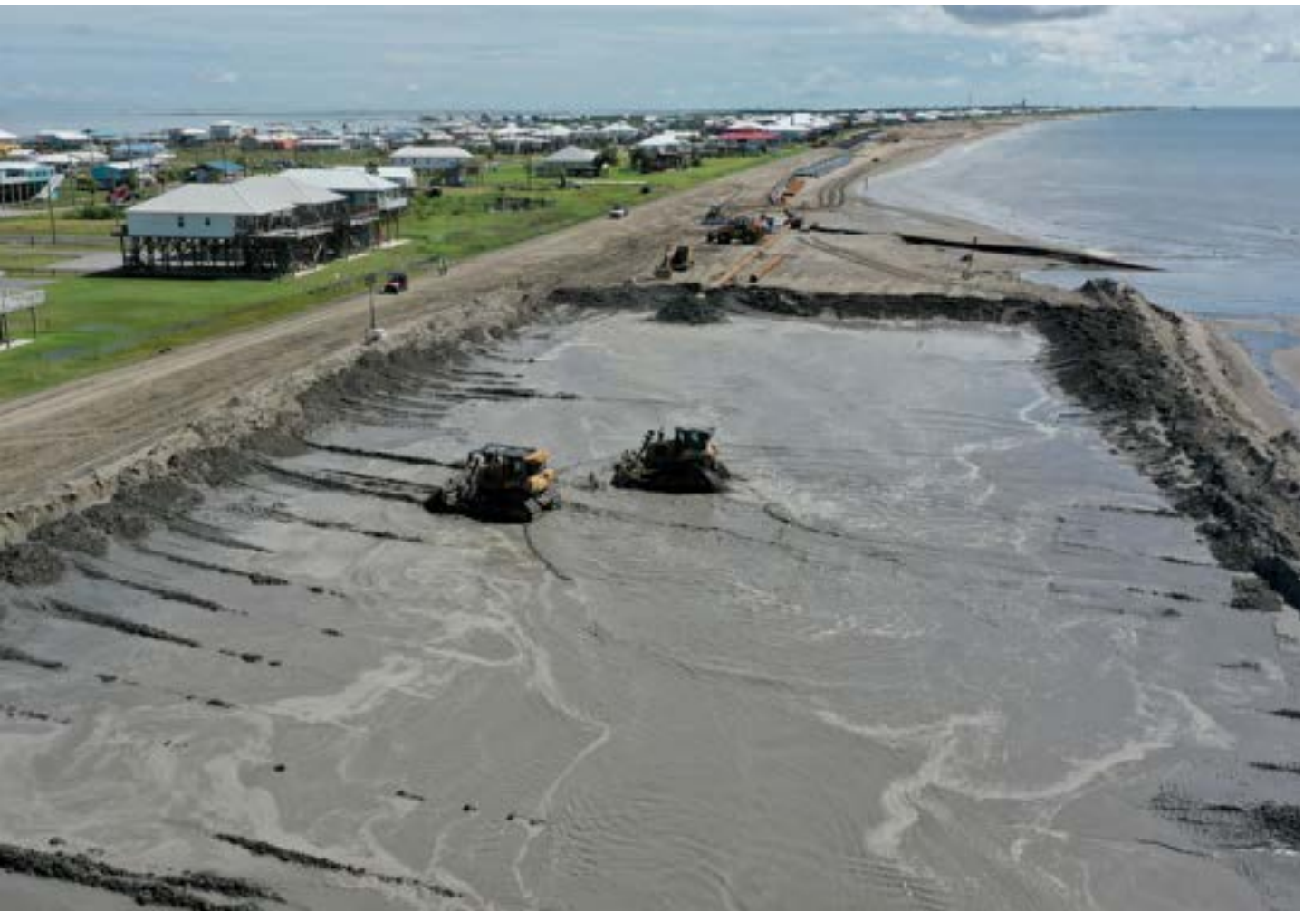
Grand Isle Dune and Beach Restoration
