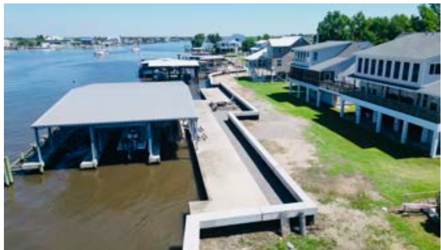
Homes along the Barataria Bayou are protected by new floodwalls
