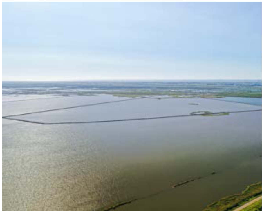
Containment dikes near No Name Bayou
